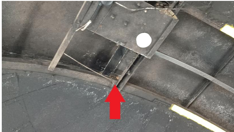
Fig. 28: Dome Aperture closing limit switch
