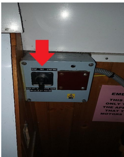
Fig. 3: Control Panel Switch Box Rotary Switch set to OFF
